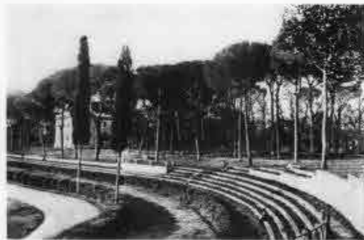
Fig. 9. Amphitheater, Villa Borghese, Rome (from Latham, Gardens of Italy ).
